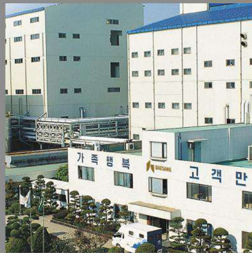
GUNSAN PLANT's General View
